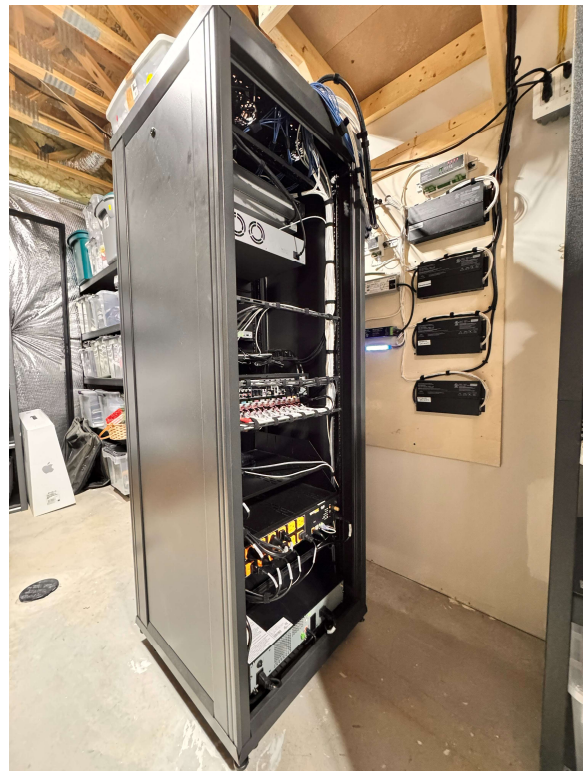
Equipment Rack Location Showing the Projector Shelf and On-Wall LED Lighting Drivers
