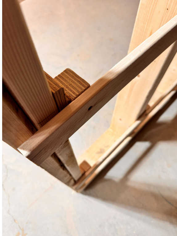
HushFrame Block Detail with Furring Strips
